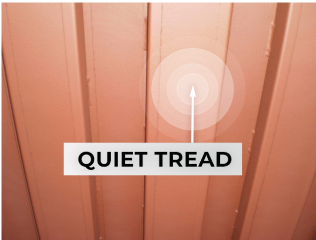
Shop applied to new landing, with primer
