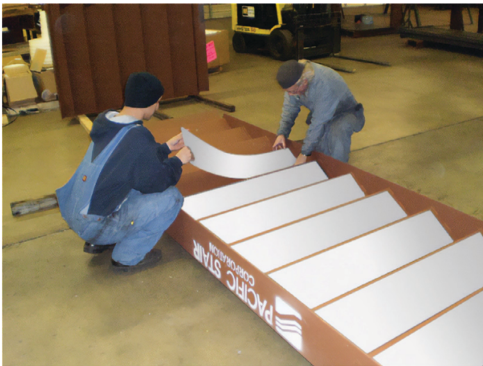
Shop applied to bottom of new metal plate stairs
