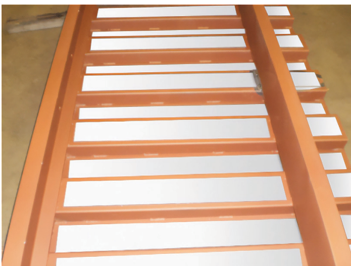
Shop applied to bottom of new metal landing
