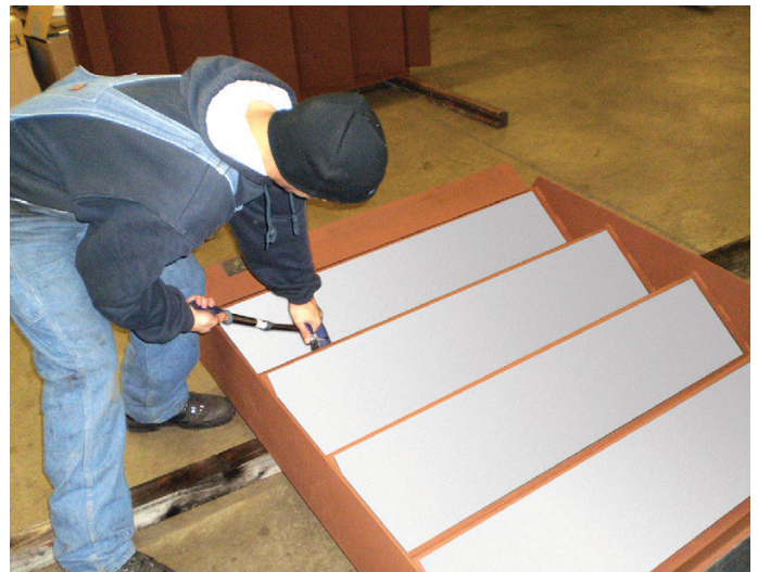
Using a commercial-grade vinyl roller
